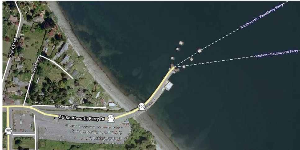
Figure 14 – Aerial view of the WSF ferry terminal at Southworth, WA
